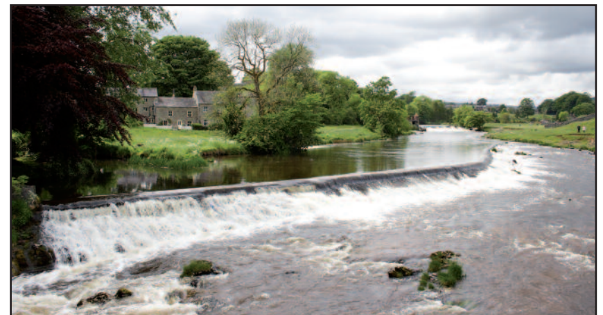
The weirs near Linton Falls.
